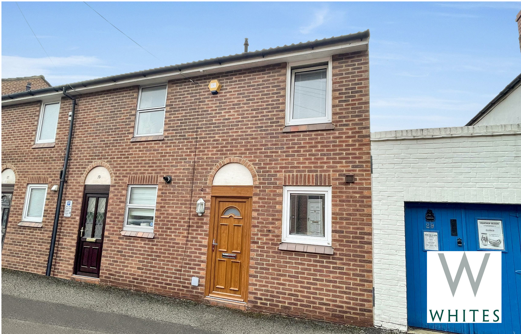
21 Greencroft Street, Salisbury, Wiltshire, SP1 1JF
